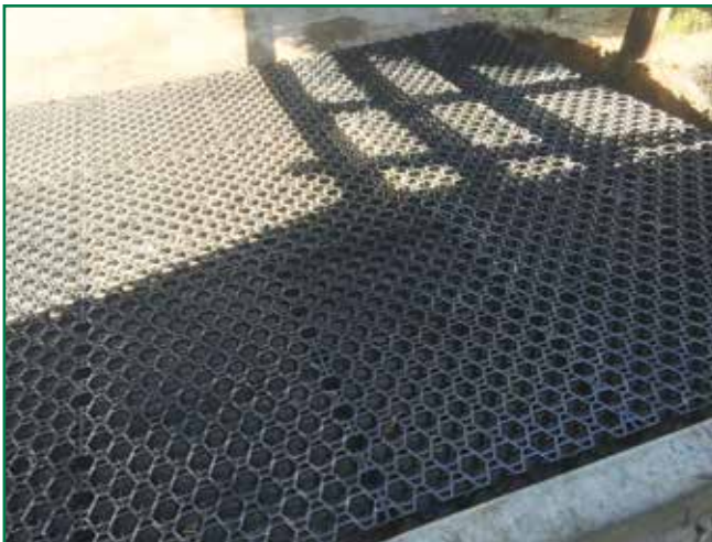
Laying Ground Cell
