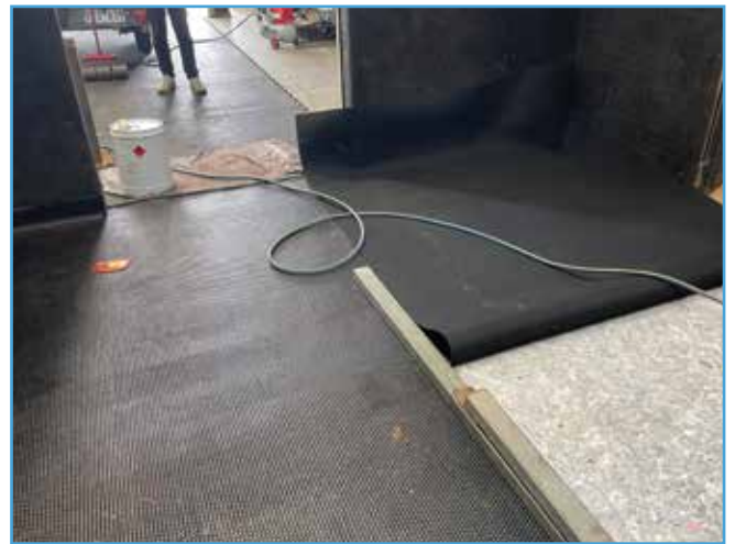
Laying of Cloth Insertion
