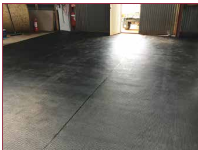
Breezeway - Hammertop Cloth Insertion
