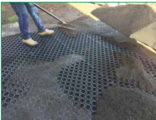
Stable Complex - Entrance
