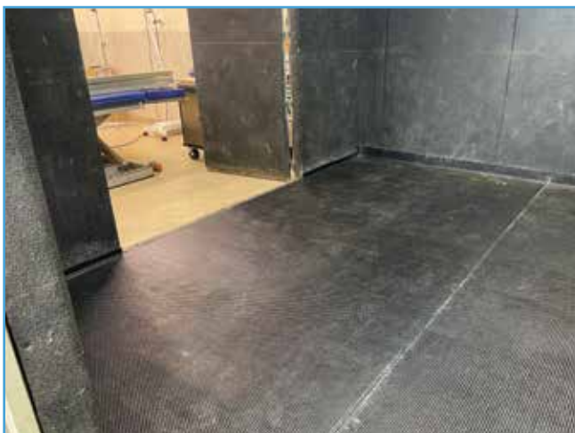
Completion of flooring
