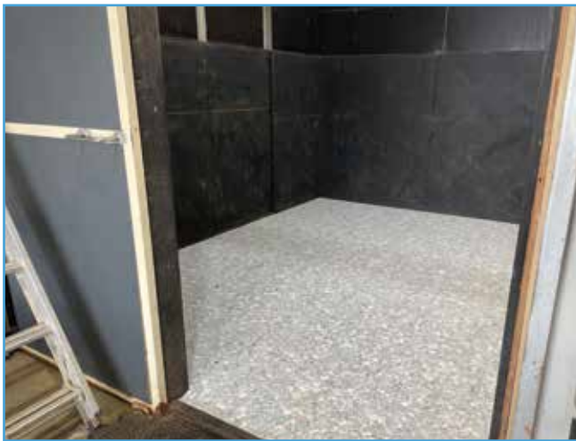
Completion of Shock Pad
