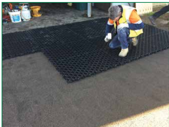
Stable Complex - Entrance
