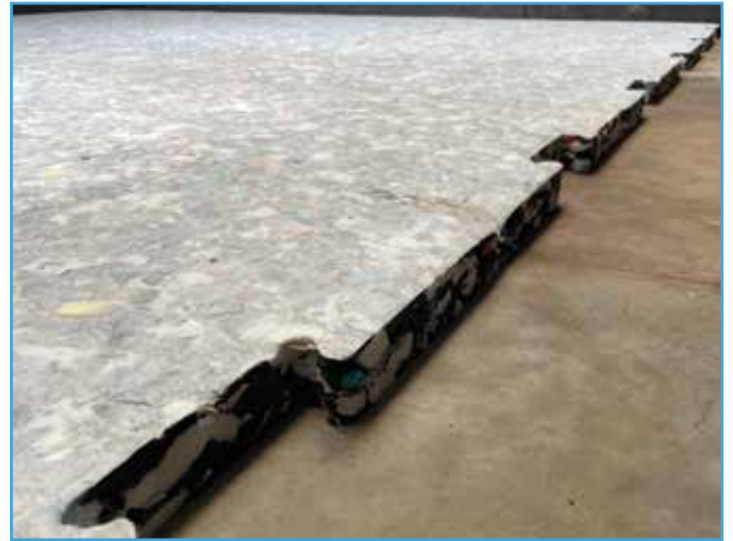
Installation of Shock Pad
