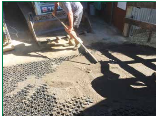
Infill of Ground Cell
